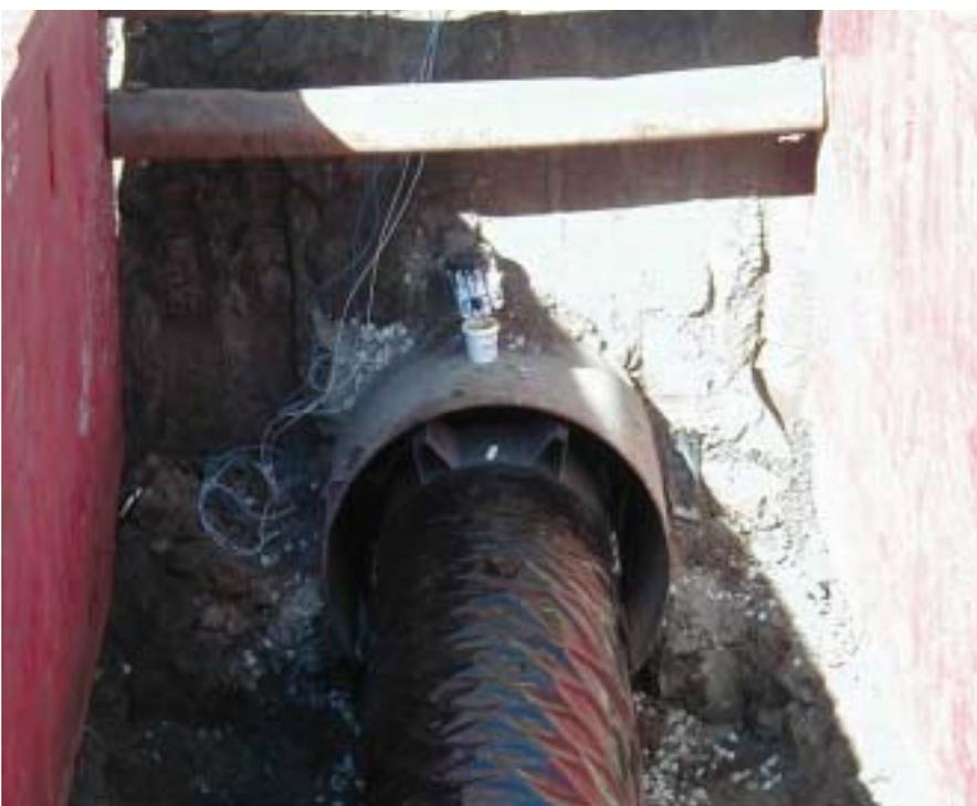
Electrical isolation in casing sleeve at road crossing.
