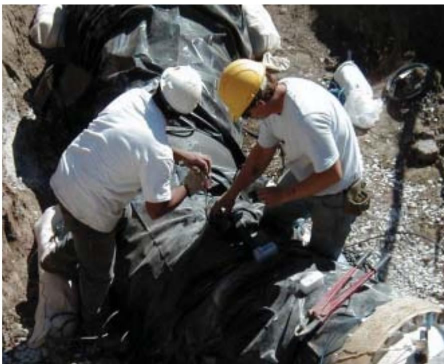
Connecting cable bonds using exothermic welding.
