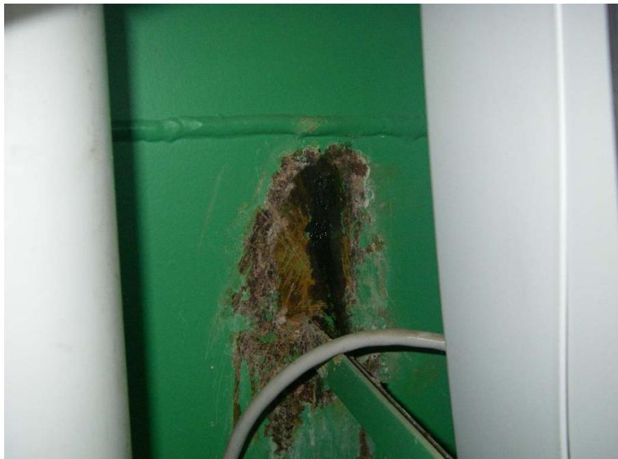
Figure 2 – Corrosion Perforation of Pump Station Wall
