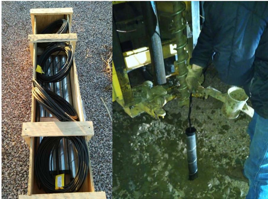
Figure 5 – Left: Crated Canistered Anodes; Right: Anode Being Installed
