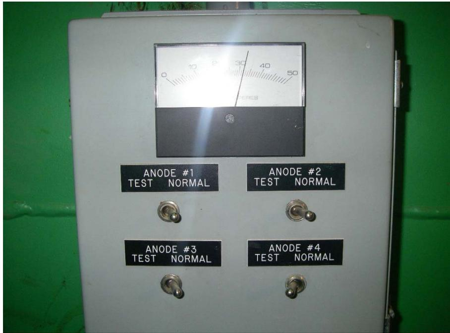
Figure 3 – Test Box for Sacrificial Anodes
