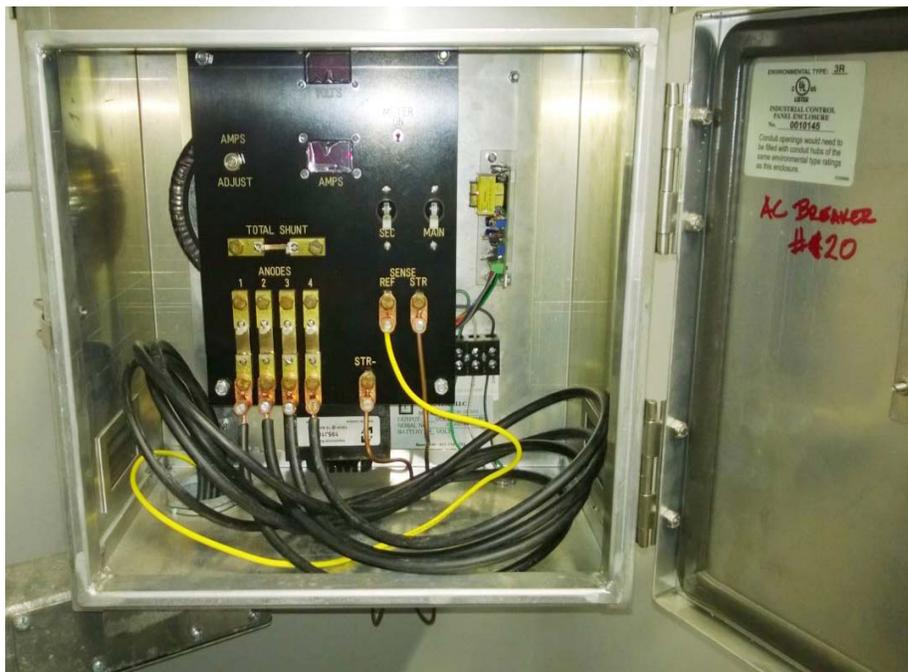
Figure 6 – CP Rectifier with Integral Anode Junction Box
