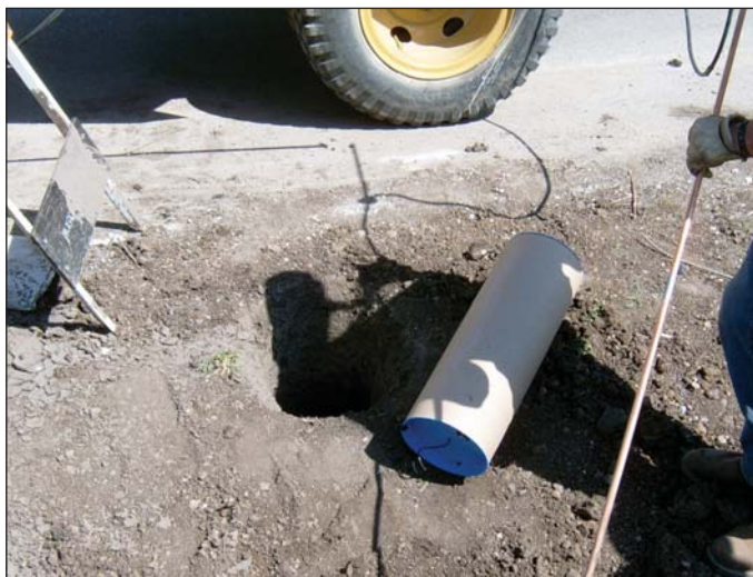
Once the stud is attached and the weld verified as secure, the prepackaged sacrificial anode is lowered into the hole (left). After it is placed in the hole, the anode is backfilled with limestone fines, native soil, and water (right).
