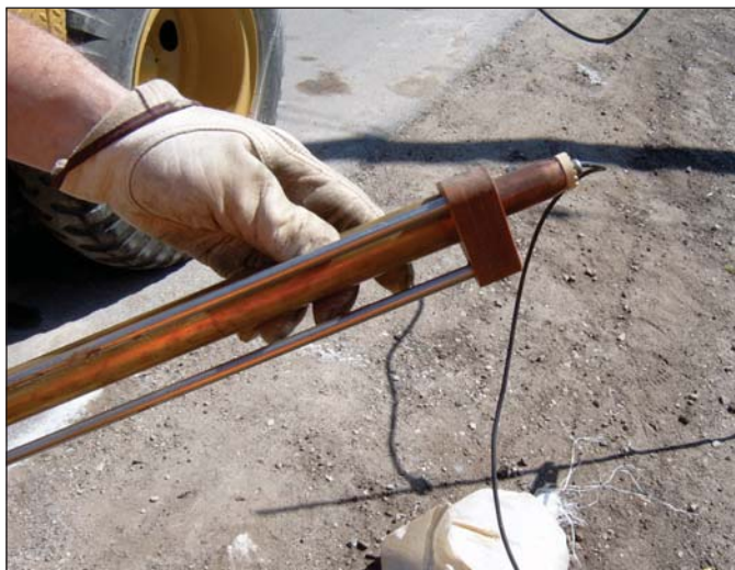
After an anode borehole is drilled and the remaining soil is removed with vacuum extraction equipment, a steel stud is welded to the top of the pipe (left). The stud fits into the end of an insulated extension tool (right) that is used to allow the welder to reach the top of the pipe and contact the pipe surface.
