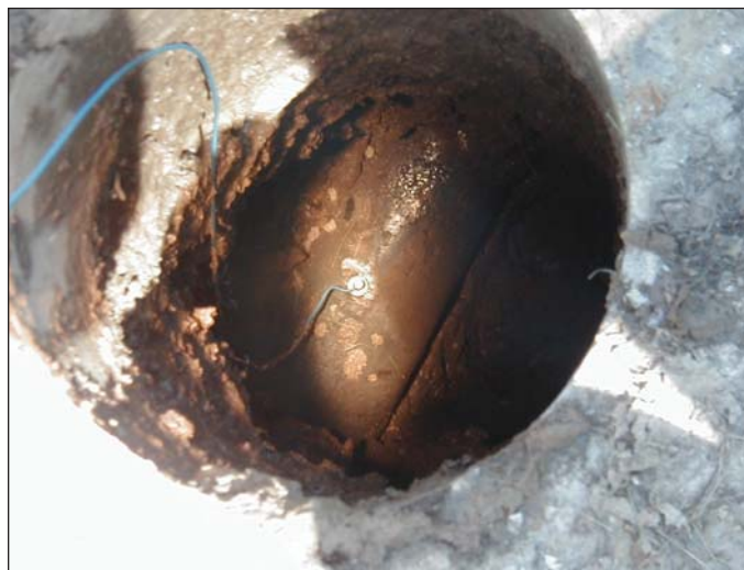
After an anode borehole is drilled and the remaining soil is removed with vacuum extraction equipment, a steel stud is welded to the top of the pipe (left). The stud fits into the end of an insulated extension tool (right) that is used to allow the welder to reach the top of the pipe and contact the pipe surface.
