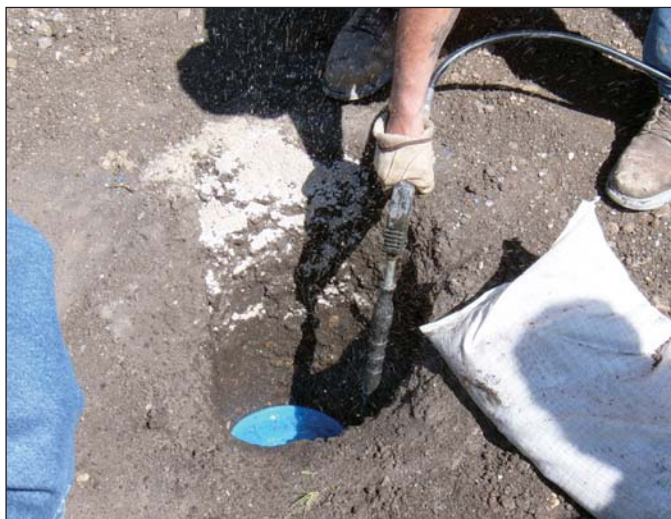
Once the stud is attached and the weld verified as secure, the prepackaged sacrificial anode is lowered into the hole (left). After it is placed in the hole, the anode is backfilled with limestone fines, native soil, and water (right).
